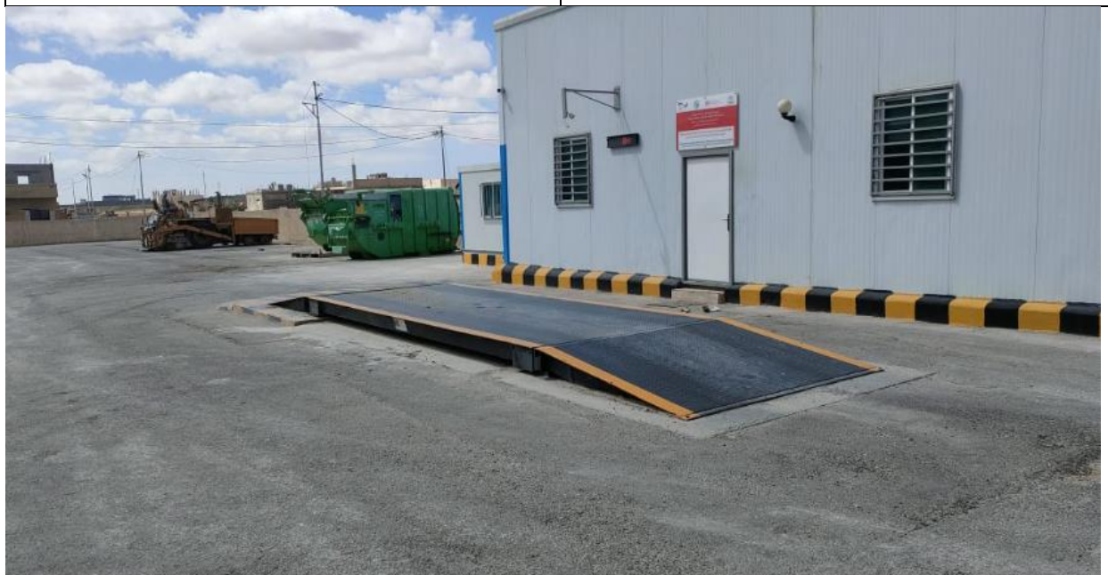
Figure 12 Weighing Bridge with a capacity of 15ton.
